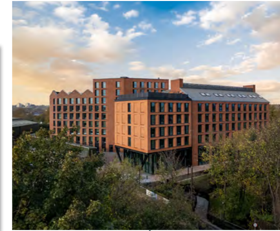
Sunday Mills Completion
