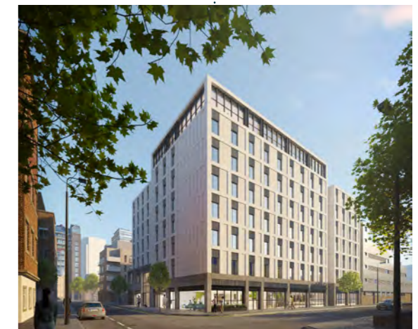
Florence Dock, Battersea Completion
