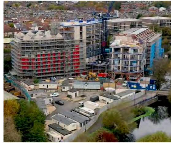
Sunday Mills Start on site
